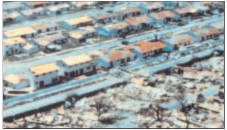
After Hurricane Andrew, photos taken in several parts of south Florida showed homes on one side of a street completely destroyed, while homes on the other side suffered minimal damage. In many cases, construction techniques for the heavily damaged buildings were well below the minimum standard required by the adopted building code.
