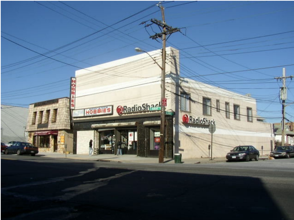
FRONT OF BUILDING
