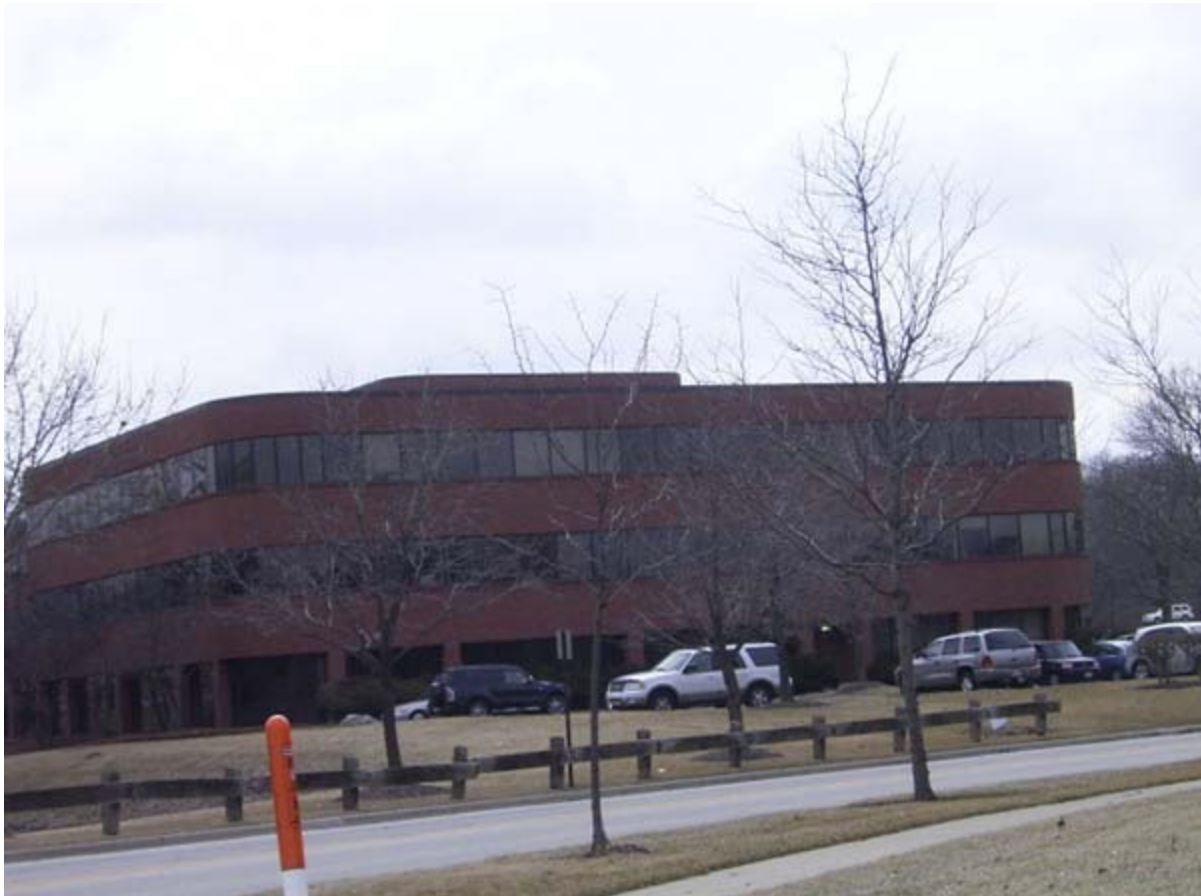
FRONT OF BUILDING
