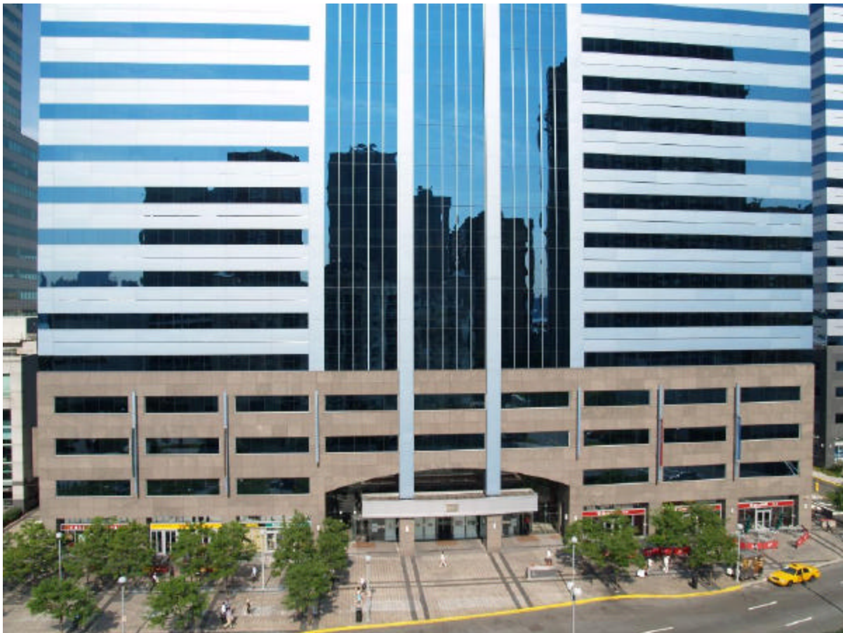
FRONT OF BUILDING
